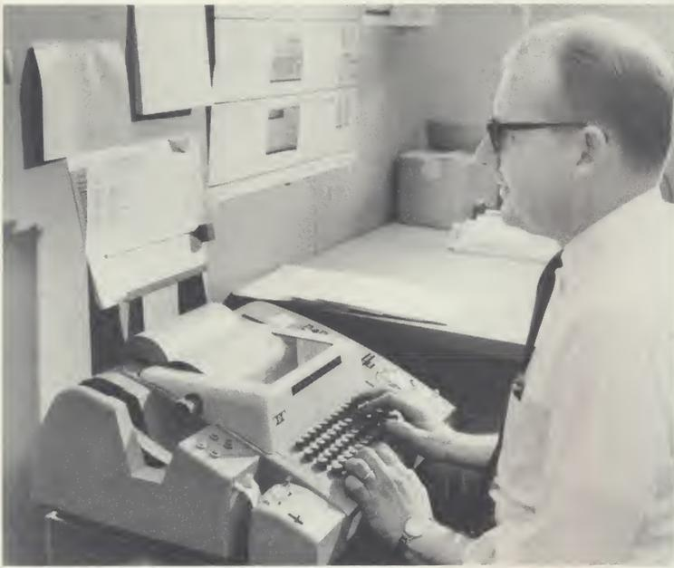
Engineers and scientists at Appliance Park communicate directly with the computer via a Teletype Model 33 ASR (automatic send-receive) set. The "conversation" is recorded as page copy, but a paper tape can be punched simultaneously. Shown here is Stuart R. Kunz, Specialist Engineering, Merchandized Information Systems.
