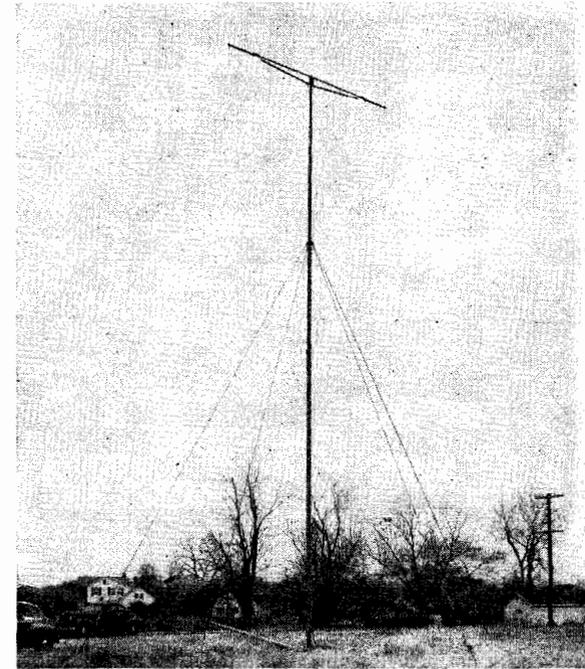
FIGURE 1.—Antenna assembly, 75-foot plywood mast, two dipoles on spreader boom, and erector boom at side near ground, of the Models SCR-573-A and 574-A.
