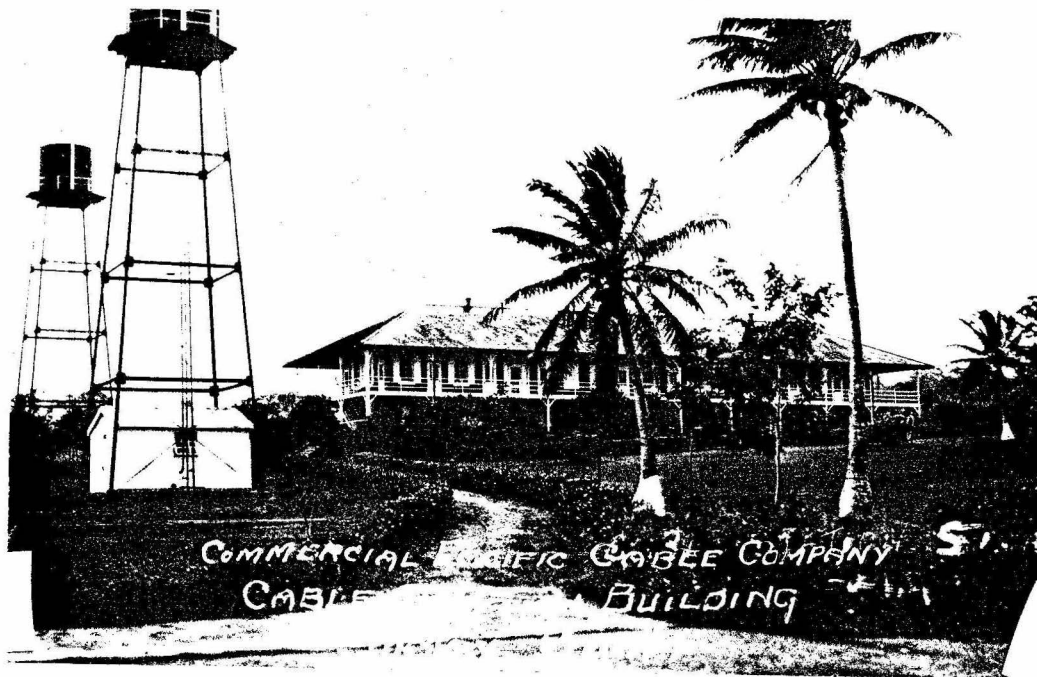
Cable station, Sumay, Guam 1935.
