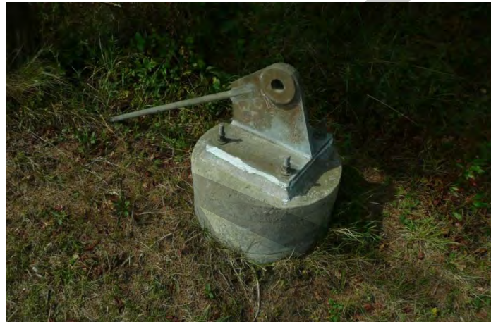
NORD antenna anchor base. The rod extending into the ground has either an earth screw or buried concrete block. The insulated radiator wire is shackled to the eye of the anchor.
